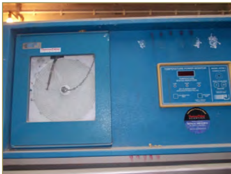
Defunct temperature recorder on a BSU in Sagardighi RH - Murshidabad
